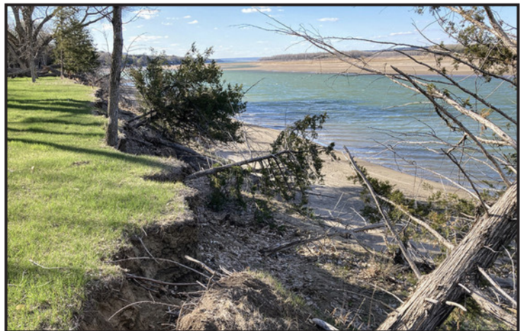
Several more cedar trees collapsed along our eroding river bank after a winter with heavy snowfall in 2022-23. Trees often take chunks of land down with them. The river is usually quite low in early spring. Looking upriver toward exposed sandbars, April 30, 2023.
